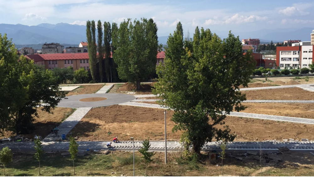
During the construction of the City Park in Gjakova
